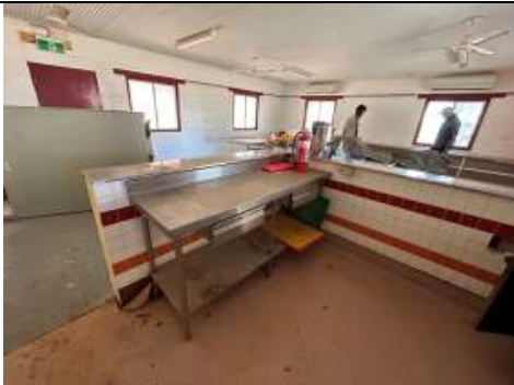
Photos Showing Current Condition of Wutungurra Womens Centre:
