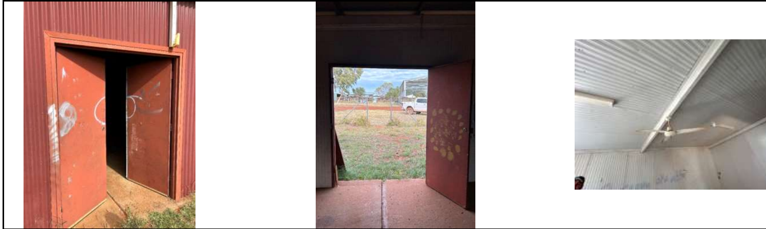
Photos Showing condition of Epenarra Men's shed before Refurbishment Project
