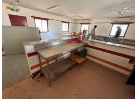
Photos Showing Current Condition and Upgrades of Wutungurra Womens Centre:
