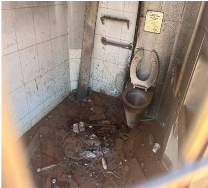
Photos: Current condition of Toilet block
