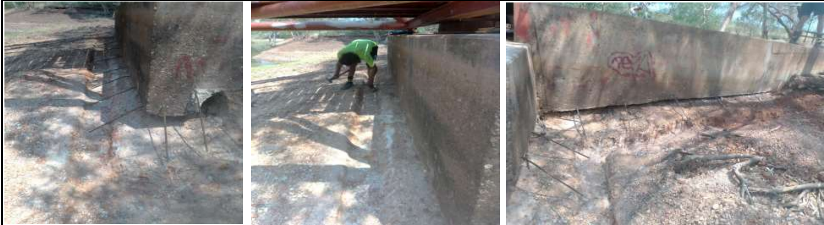
Photos: Before and After for the footings
