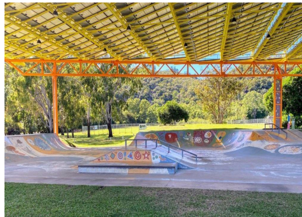
SOLAR POWERED SKATE PARK WITH SHADE STRUCTURE - SUITABLE TO POWER THE WHOLE PURKISS PARK - EXAMPLE IS MAGNETIC ISLANDS SKET PARK
