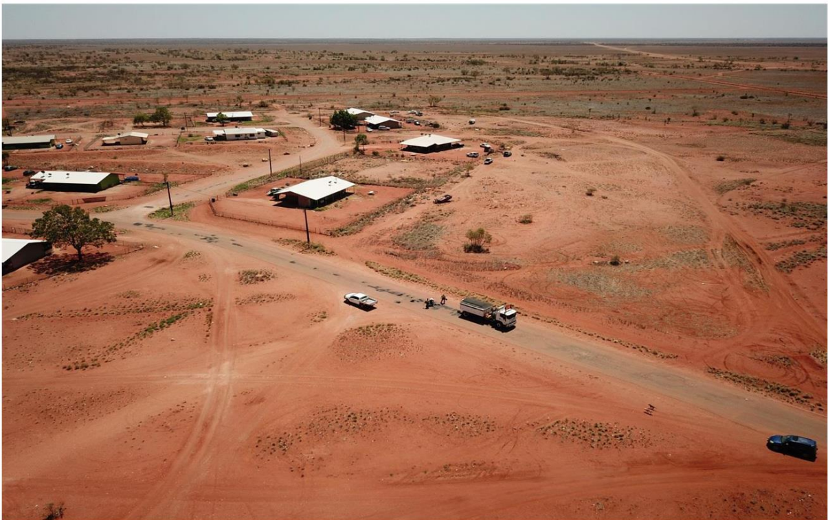
Council road crew patching using Flocon truck
