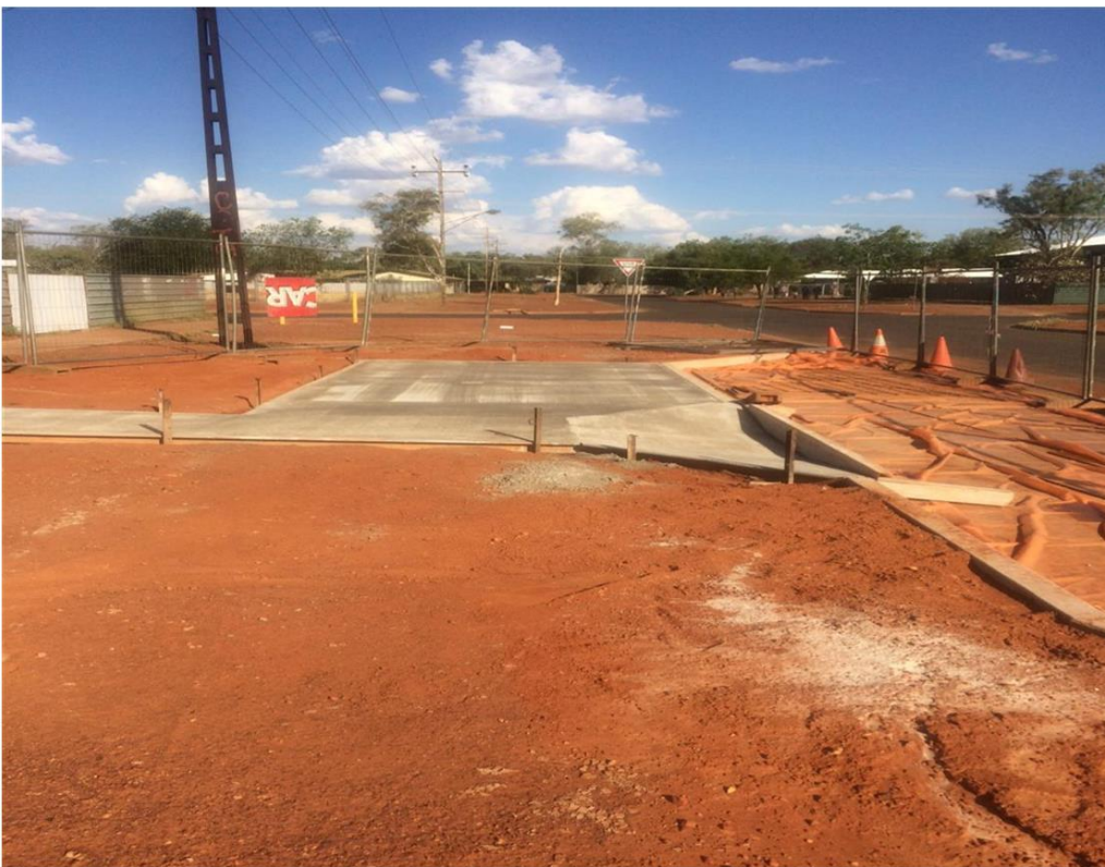
Bus shelter and bay construction Pinnacles Rd, Tennant Creek
