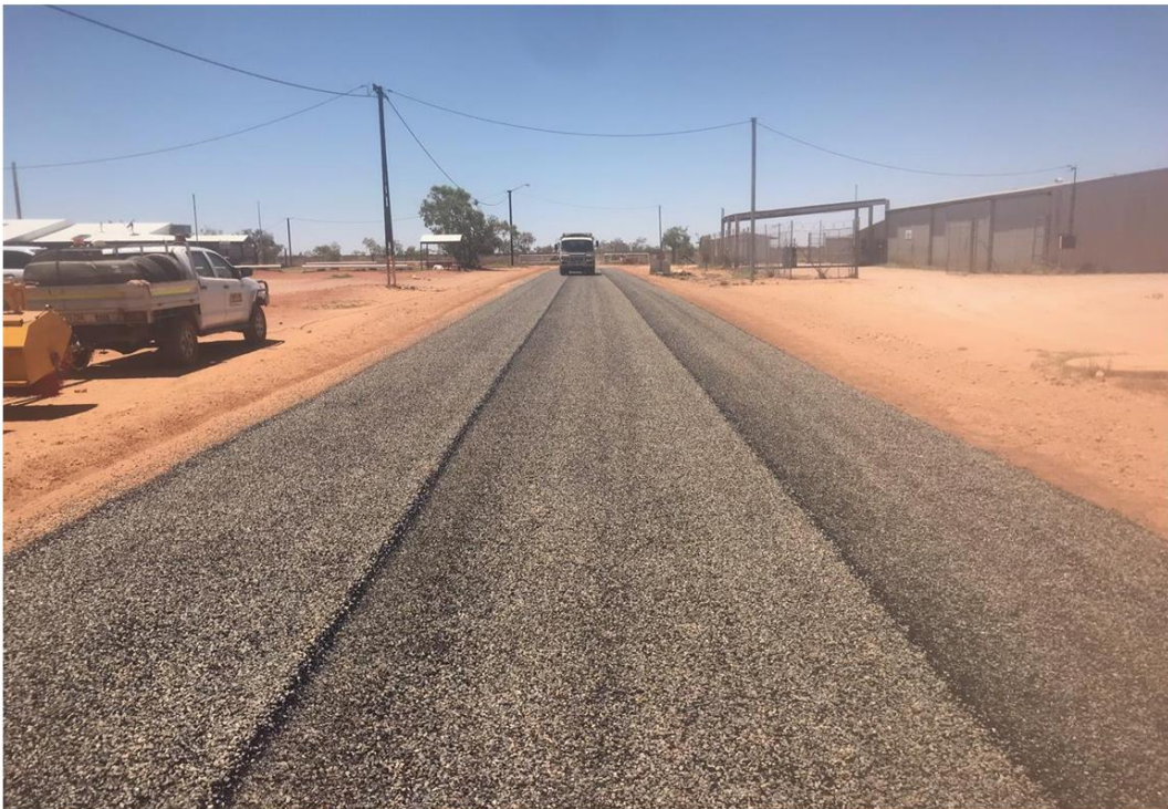
Application of 1 st seal at Antyiper St, Alpururulam
