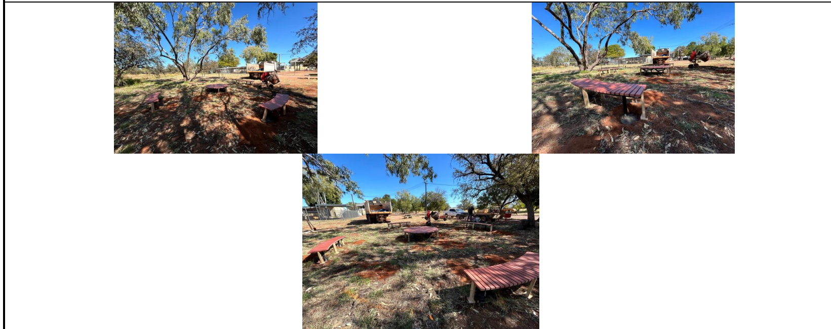
Photo Showing Elliot Yarning Circle during installation:
