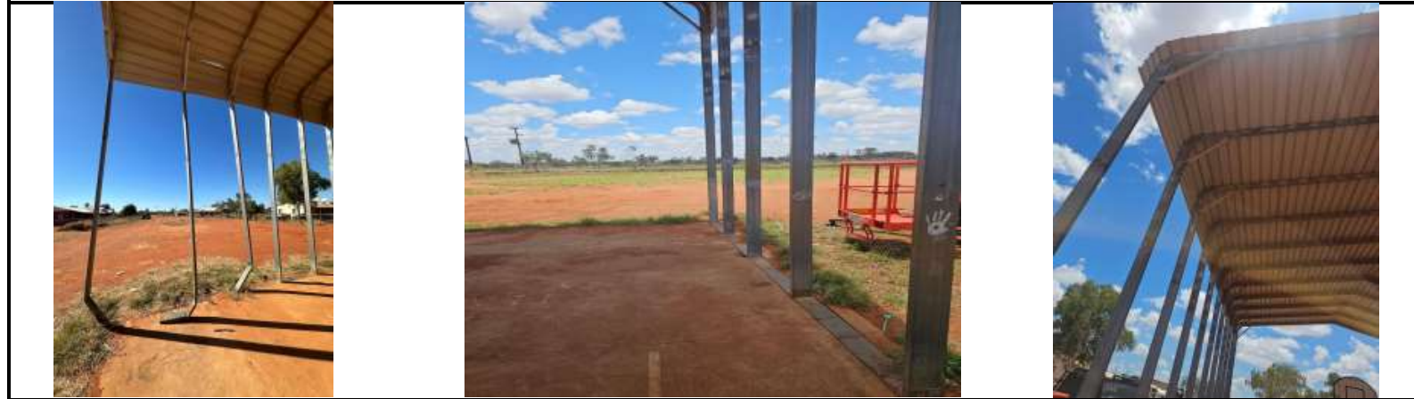
Photos Showing Condition of Basketball Court: Before and After
